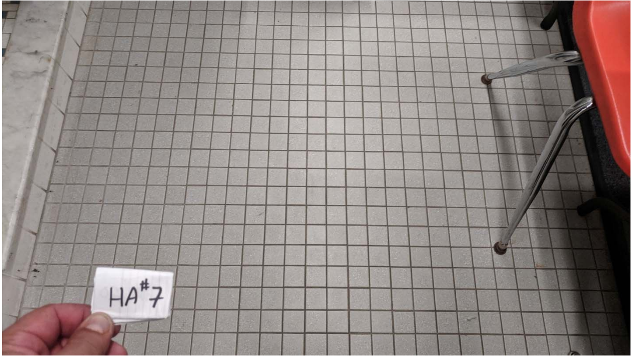
HA #7 – 2"x 2" Gray Ceramic Floor Tile Grout/Thinset
