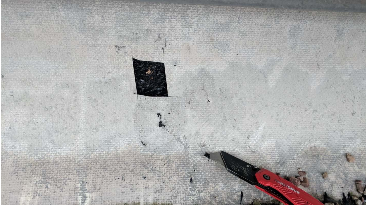
HA #28 – White Perimeter and Curb Roofing
