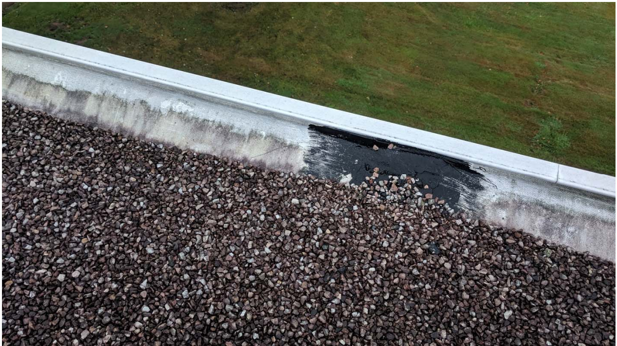
HA #21 – Black Roof Seam Mastic
