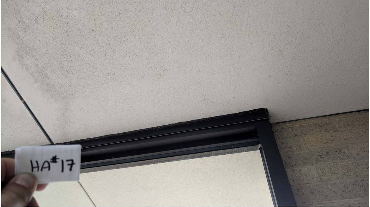
HA #17 – Brown Masonry Joint Sealant #2
