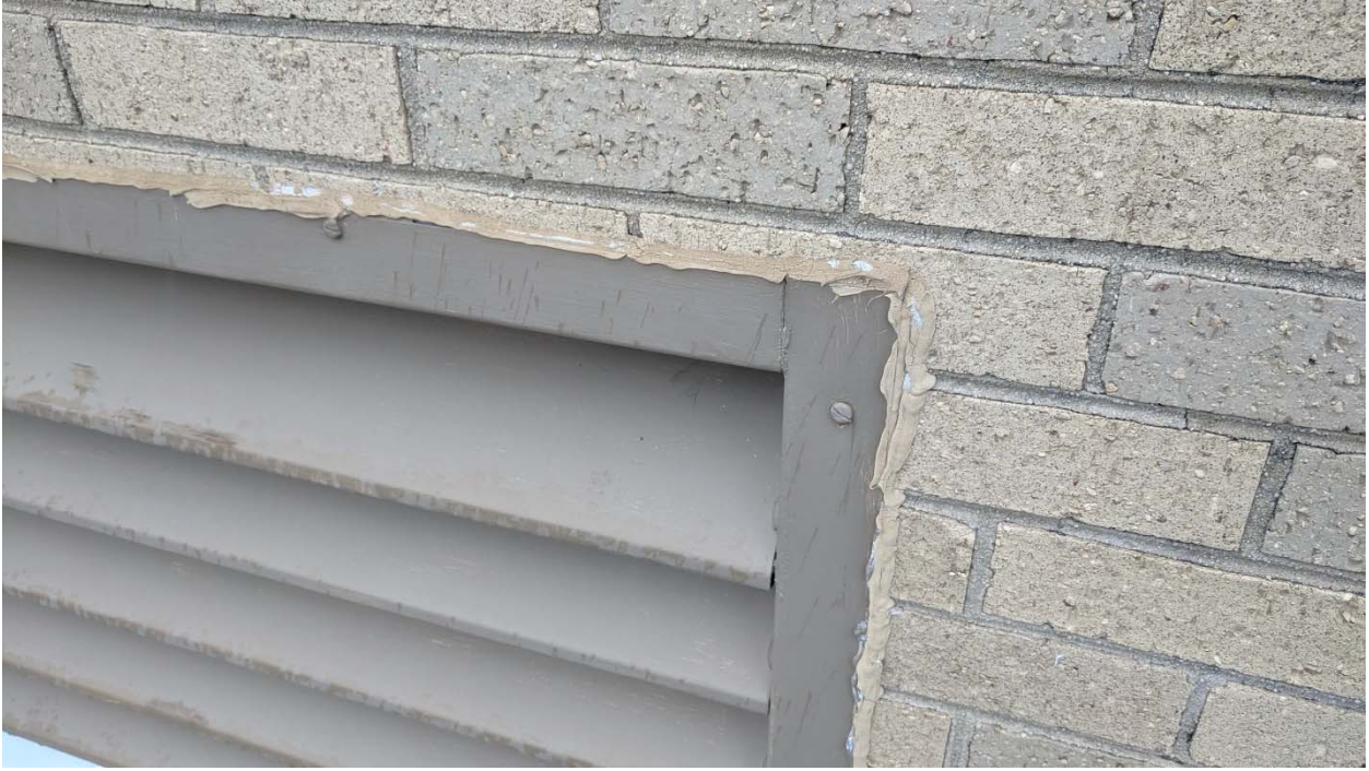
HA #22 – Tan Vent Masonry Joint Sealant
