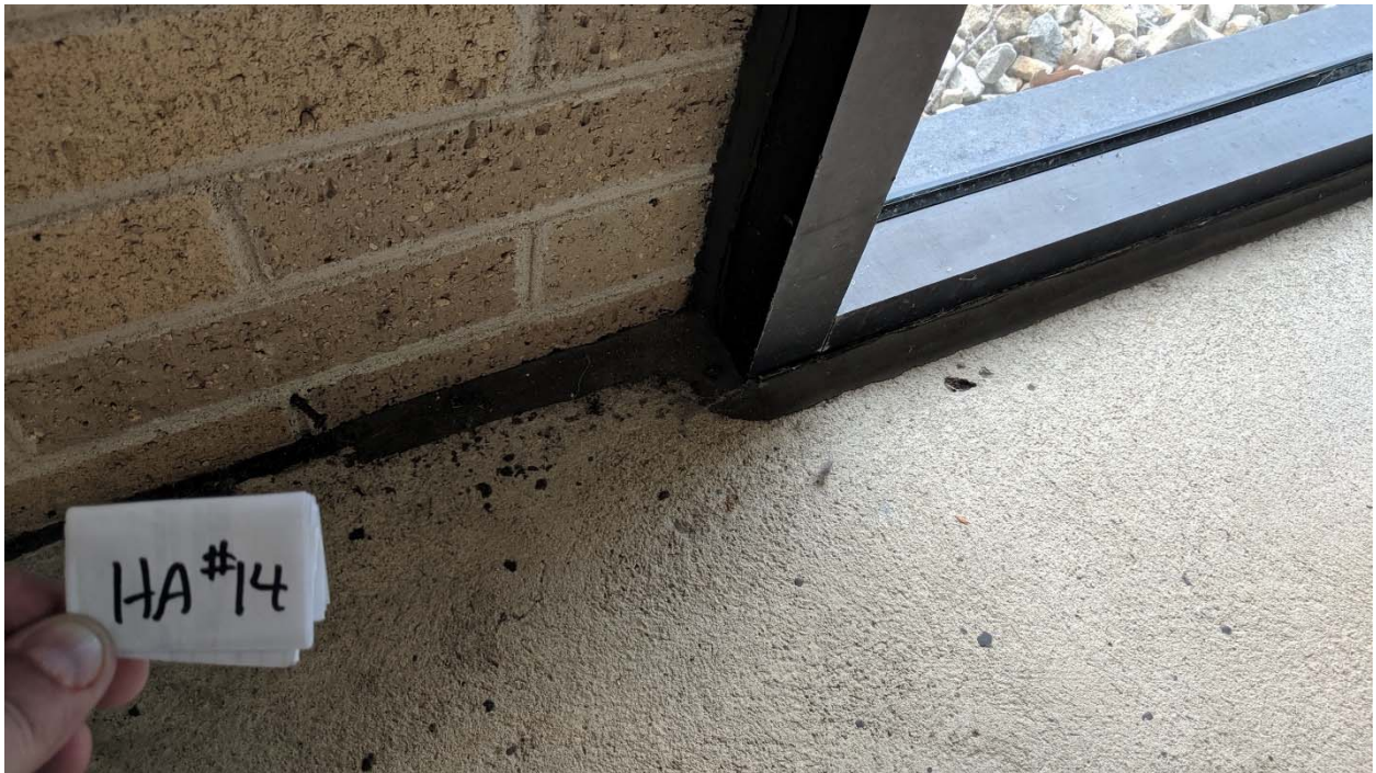
HA #14 – Brown Masonry Joint Sealant
