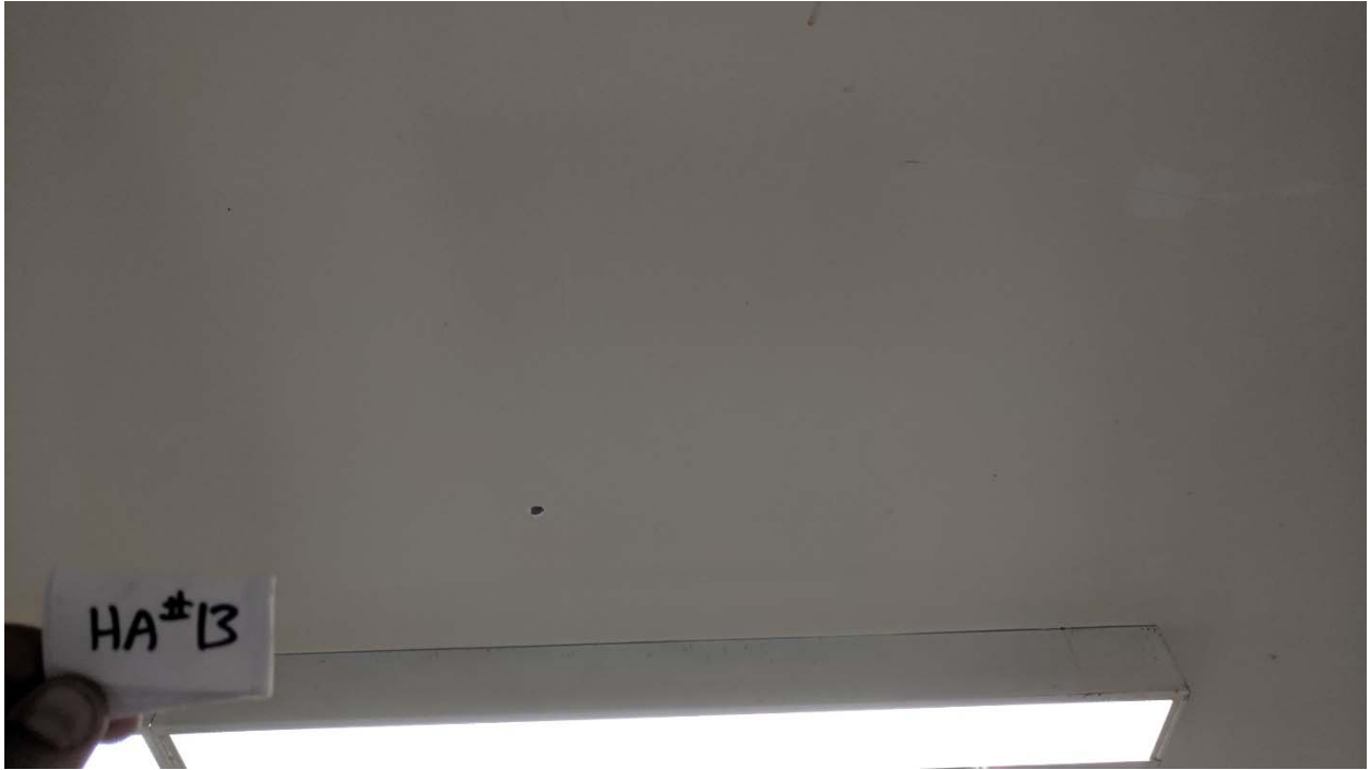
HA #13 – Finished Plaster Ceiling
