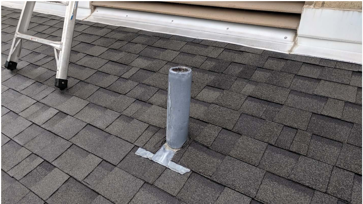
HA #25 – Black Asphalt Roof Shingles and Tar Paper
