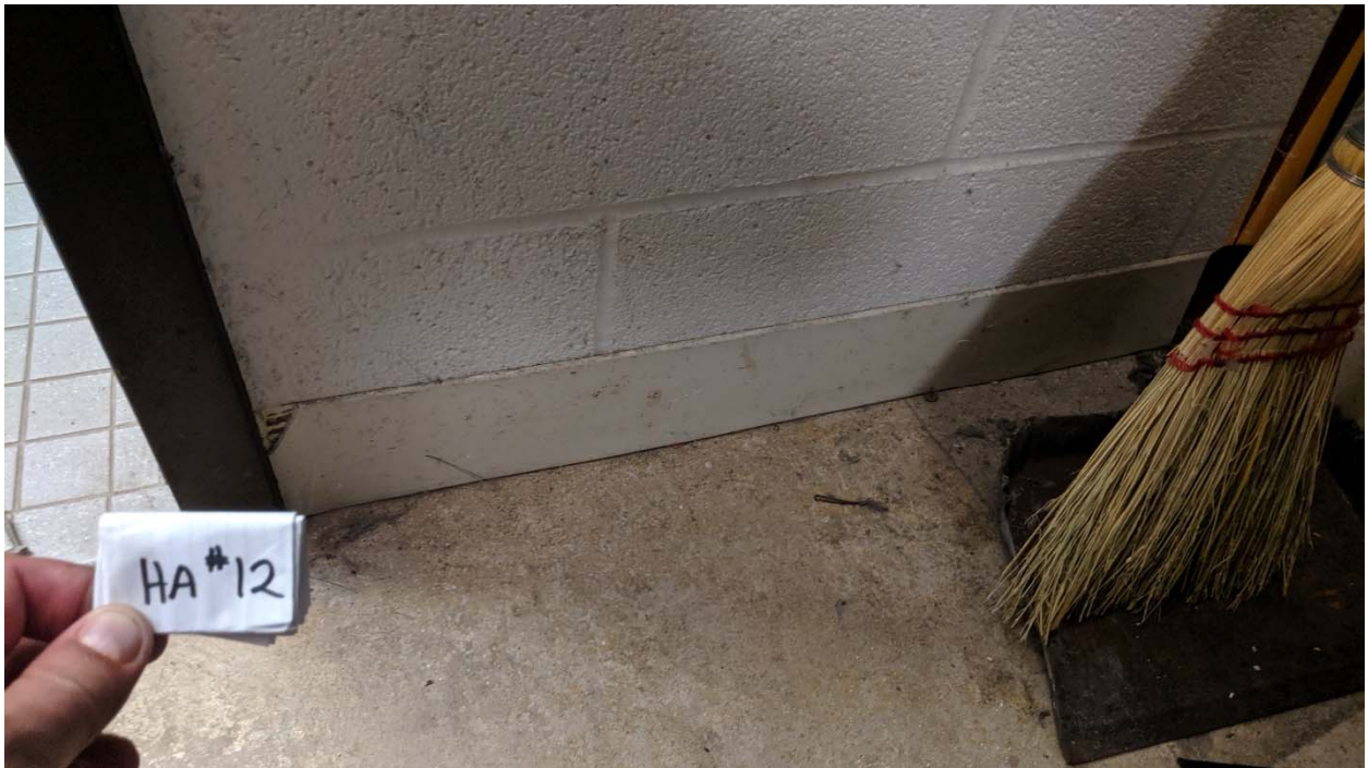
HA #12 – White Vinyl Cove Base and Tan Mastic
