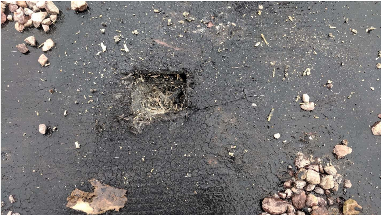
HA #27 – Black Built Up Roofing
