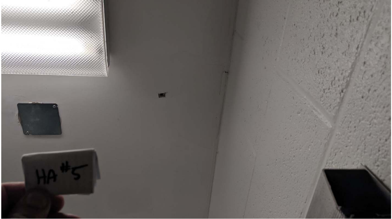
HA #5 – Gypsum Board Sheeting
